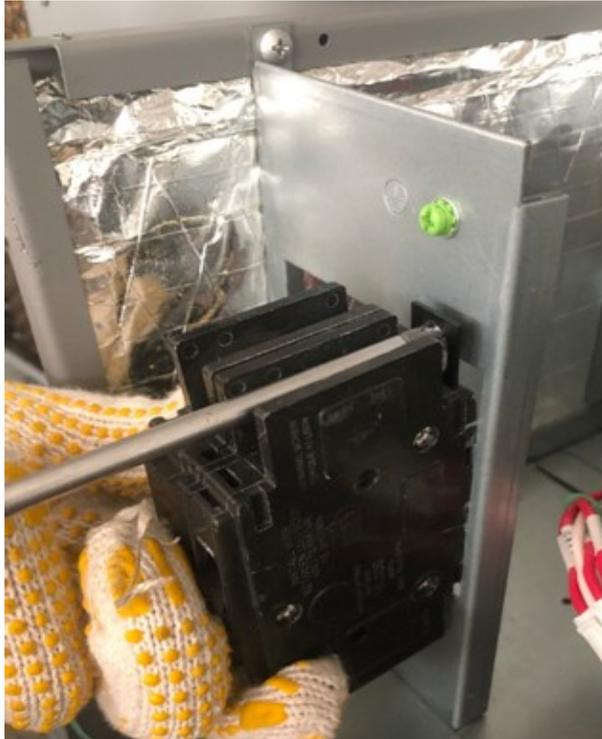
7. Disconnect line voltage from L1 and L2 terminals if applicable. Connect the electric heater terminal.
