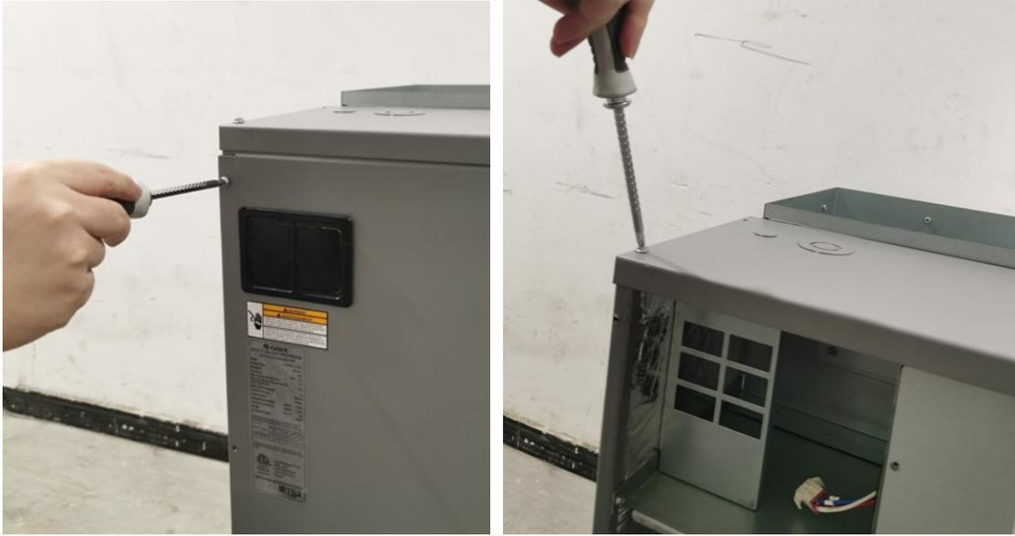
2. Disassemble the electrical box.
