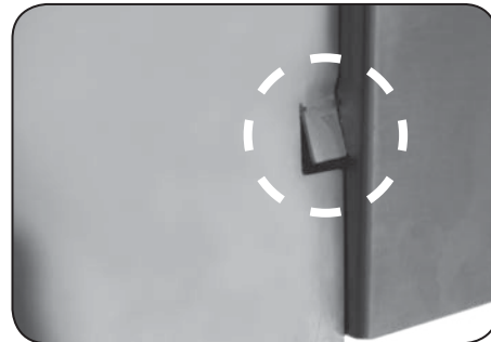
Fig. 19-2 Tab slightly bent in for clearance
