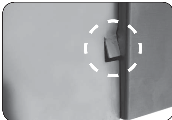
Fig. 19-2 Tab slightly bent in for clearance
