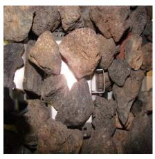
4) <u>Blowout Box:</u> Do not cover blowout box vents or opening with lava rock or glass. Incorrect media installation will cause the pilot flame to suffocate and turn off pit or delay main burner ignition.
