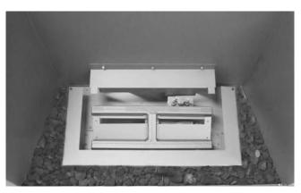
**STEP 4:** Fill around the rock platform with lava rock.Do not place lava rock on the burner tube.
