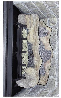
**Step (6)** Place rear log on to the log retainer 1/2" away from back of fireplace. (If refractory liner is used, make sure refractory liner is installed first then back log is to be pushed up against it as tight as possible.)
