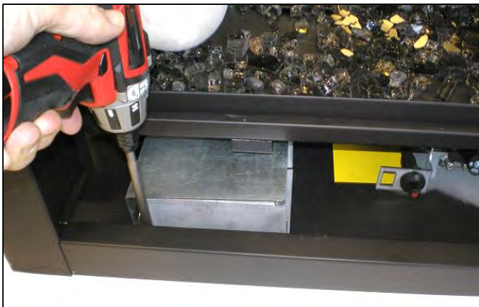
Power Vent Control Module Mounted inside fireplace.
