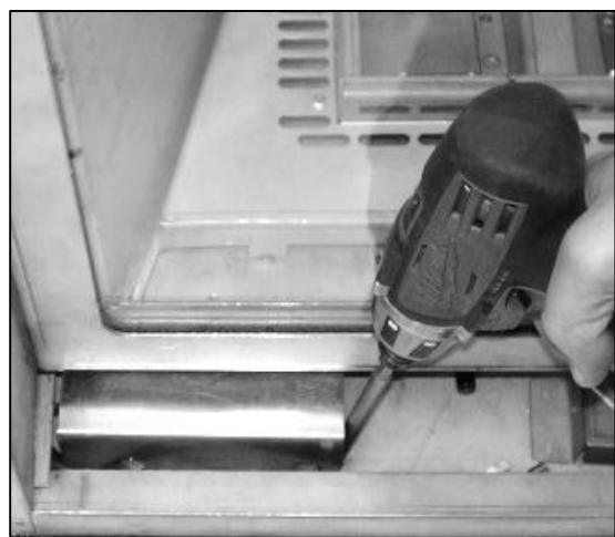
Power Vent Control Module Mounted inside fireplace.
