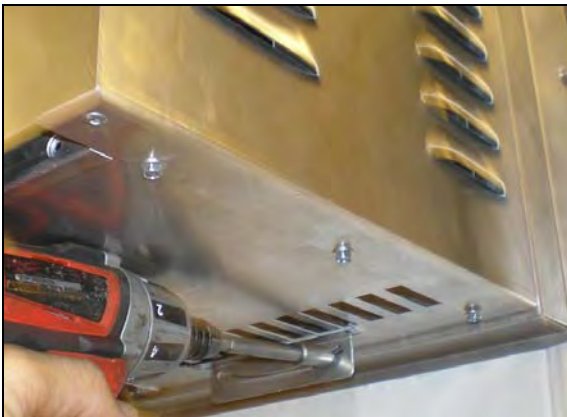
Loosen screw at bottom of Power Vent
