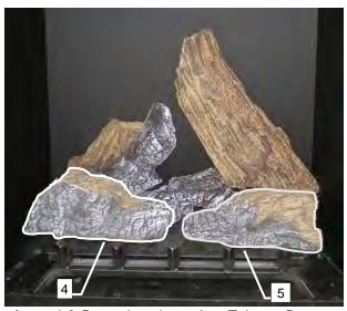
Logs 4 & 5 are placed onto Log Tabs on Burner.
