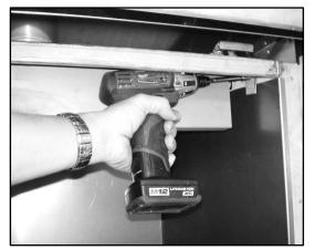
Step Four: Fix Side Liners in place using Liner Retainer Clips.
