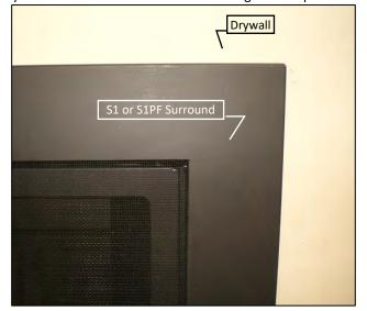
**Step Two:** Use Drywall to finish face of wall. **NOTE:** Drywall will be flush with fireplace face.
