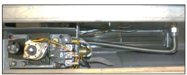
NOTE: Do not allow cords or wires to come into contact with the firebox or the underside of the burner pan.
