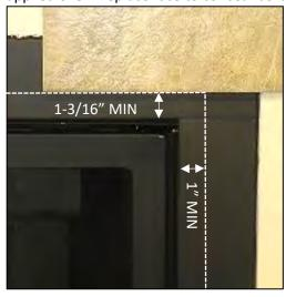
IMPORTANT NOTEL: If installing tile, brick, or other non-combustible material around the perimeter of the screen: you MUST Leave 1" of the face exposed around the fireplace opening on the Bottom and Sides, and 1-3/16" exposed on the top. This is to install and remove the safety screen. See drawings below. A Tile Lip Kit is Available. Part No. ZCV-TLK
