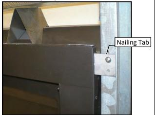
**Step Two:** Use Concrete Board to cover fireplace face. **NOTE:** Optional ZCV-TLK Tile Kit is available. Maintain clearances shown. See bottom drawings also.
