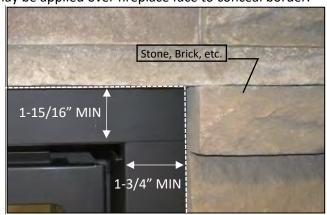
If installing stone, brick, or other non-combustible material around the perimeter of the surround: you MUST Leave 1-3/4" of the face exposed around the fireplace opening on the Bottom and Sides, and 1-15/16" exposed on the top. This is to install and remove the surround. See drawings below. A Tile Lip Kit (ZCV-TLK) is available.
