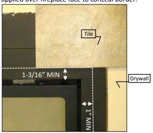
**IMPORTANT NOTE!:** If installing tile, brick, or other non-combustible material around the perimeter of the surround: you MUST Leave 1" of the face exposed around the fireplace opening on the Bottom and Sides, and 1-3/16" exposed on the top. This is to install and remove the surround. See drawings below. A Tile Lip Kit (ZCV-TLK) is available.
