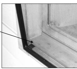
Push top of screen up against fireplace and hook onto screws in side frame. Push down on screen to lock in place.
