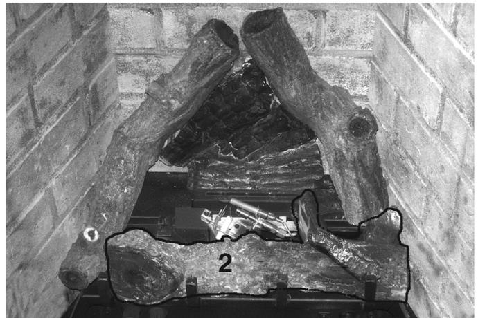
2. Locate the two notched areas of Log #2 and line them up with the two grate bars as shown.
