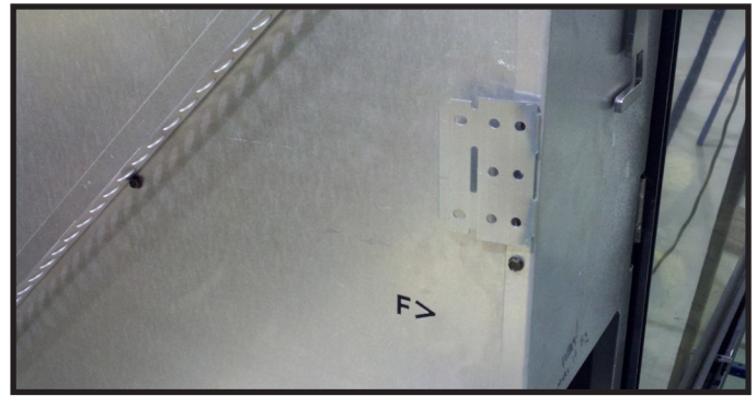
Figure 6.3 Side Nailing Tab in Shipping Position
