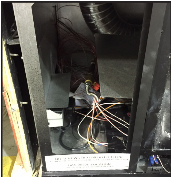
Figure 8.1 Junction Box Access
