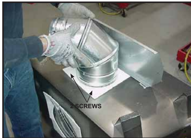
Figure 6.11 To attach the first section of vent pipe, make sure to use the fiberglass gasket to seal between the first vent component and the outer fireplace wrap. Use 2 self tapping screws to secure the gasket to the outer wrap.
