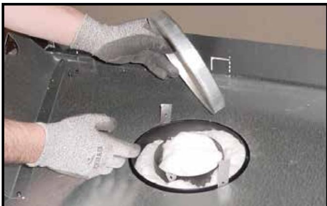
Figure 6.3 (Generic Fireplace Shown) Remove the seal cap.
