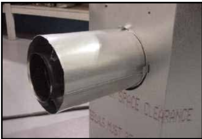
Figure 6.10 (Generic Fireplace Shown) Attach the first vent section (it will snap into place). Slide the insulation gasket (shipped in the manual bag) onto the vent section, up against the appliance and over the tabs.
