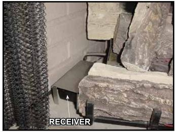
Figure 5. Receiver Location-Left Side of Log Set
