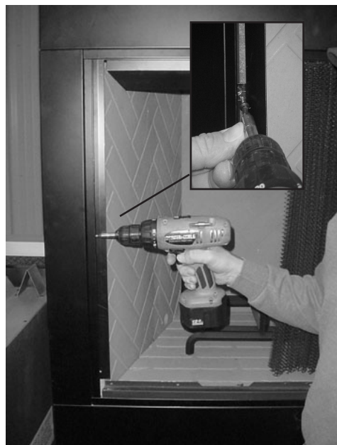
Figure 5 - Fastening the Side Filler
