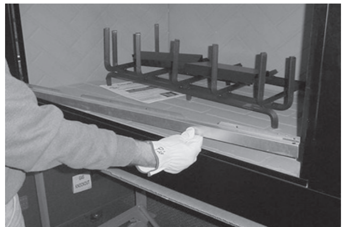
Figure 1 - Install the Door Track
