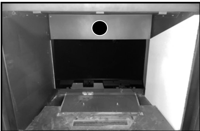
Figure 8 Rear Glass Panel and Side Insulation Board Installed
