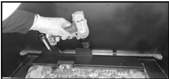
Figure 3 Install Back Refractory Support
