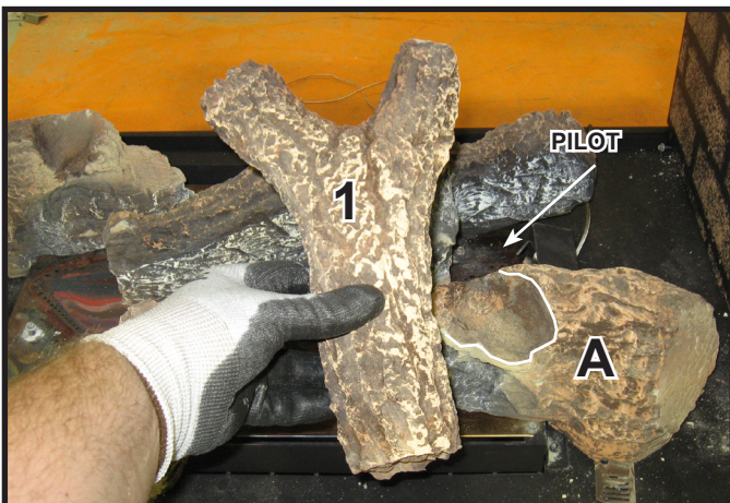
Figure 3. Placement of Log #1
