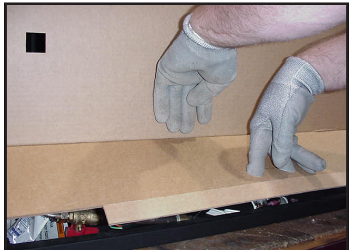
Figure 11.9 Opening Lower Access Panel
