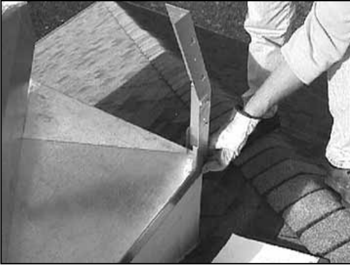
Figure 7 Secure the Legs - Side of Chase Top
