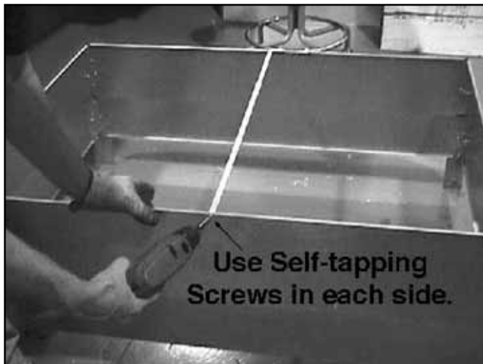
Figure 21 Attach Top Wind Brace to Shroud
