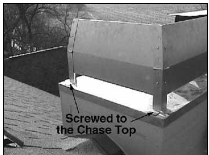
Figure 19 Shroud Attached to Top of Chase
