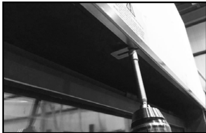
Figure 10.5. Install Trim Ring
