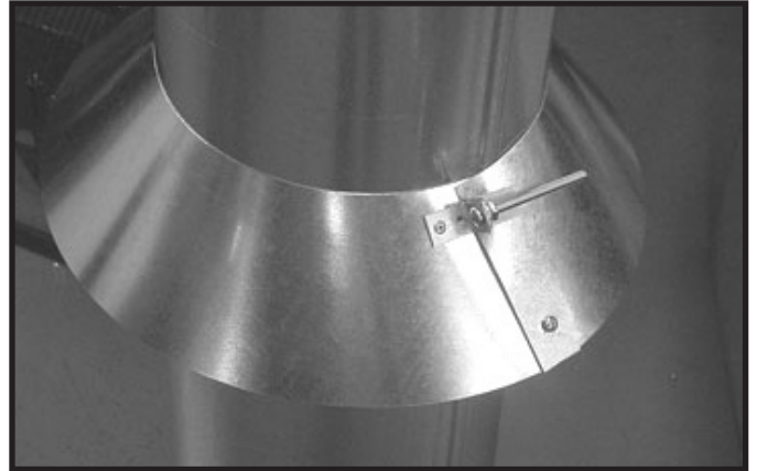
Figure 7.12 Insert Bolt into Brackets
