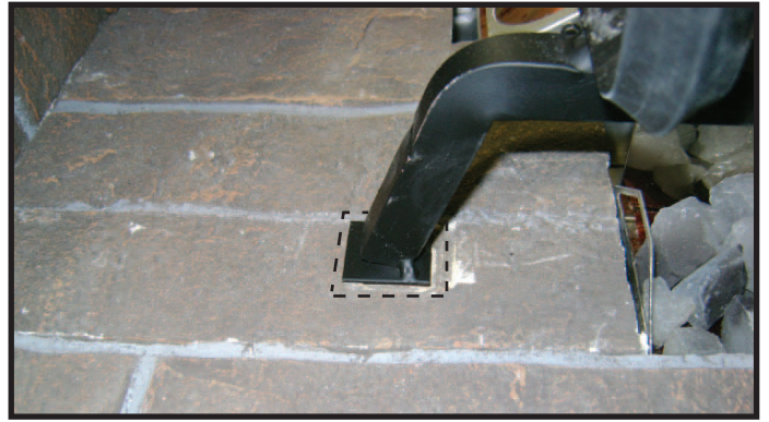
Figure 3. Grate leg placement.
