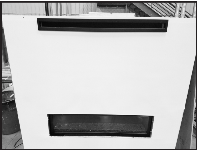
Figure 6 Vent Cover Installed
