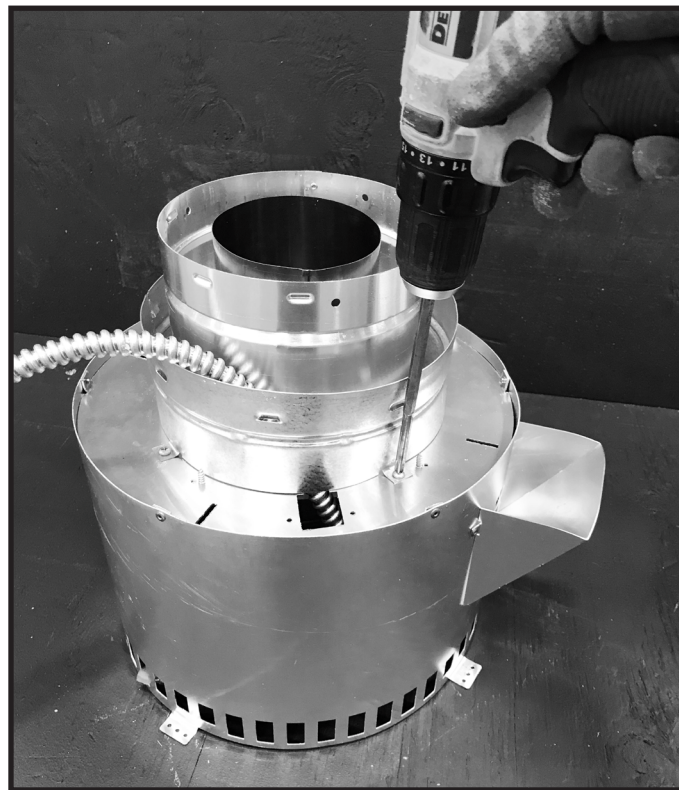
Figure 3.11 Attach Starting Collar
