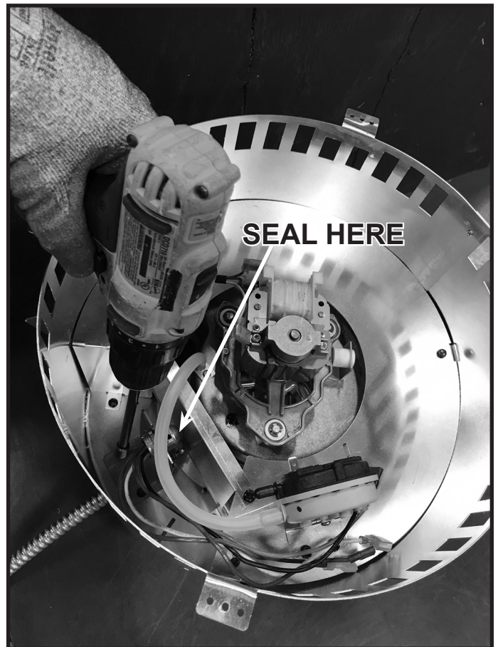
Figure 3.13 Attach Wire Harness Bracket to Bottom Dish
