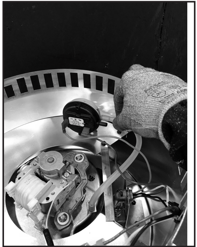
Figure 5.2 Remove Teflon Tubing
