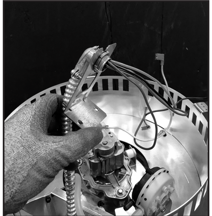
Figure 3.12 Attach PVI Wiring Harness to Bracket
