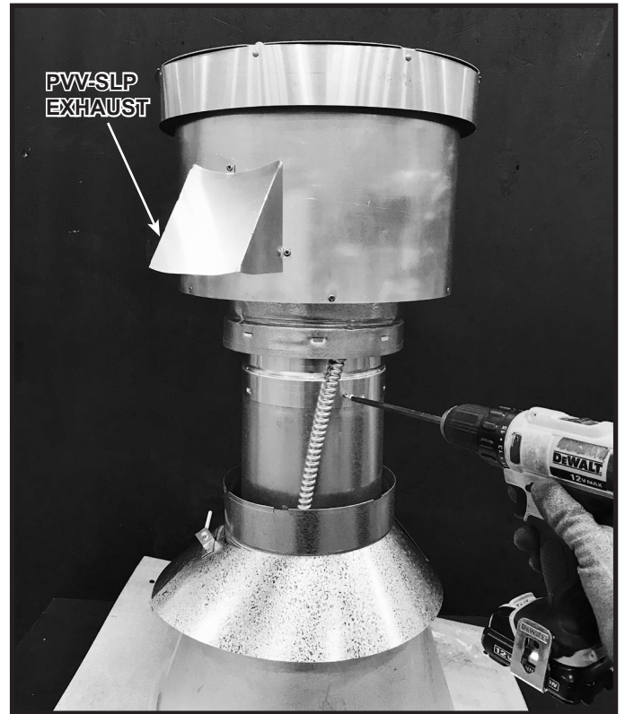
Figure 3.21 Attach PVV-SLP to SLP Pipe
