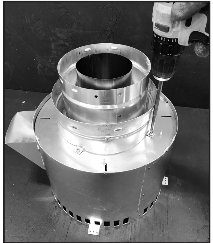
Figure 3.8 Remove Screws from PVV-SLEEVE Starting Collar
