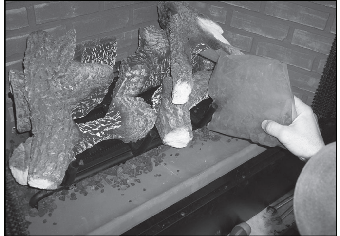
Figure 14.21 Placement of Lava Rock
