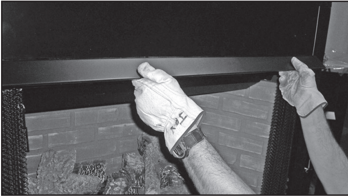
Figure 14.27 Installing the Hood
