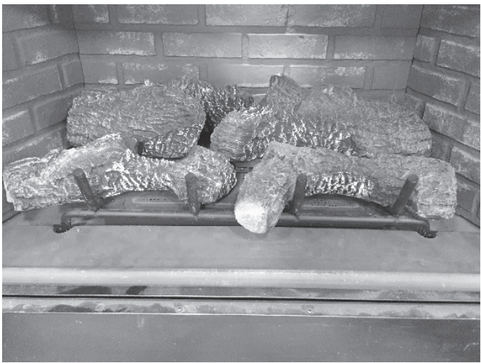
Figure 14.13 Left and Right Front Log Placement
