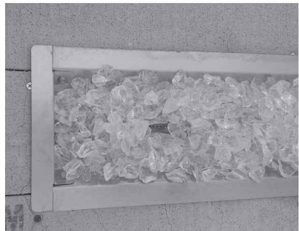
Figure 5.3 Pan Installed on Top of Finish Material
