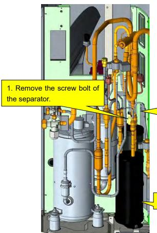
2. Remove the screw bolt of the separator.
