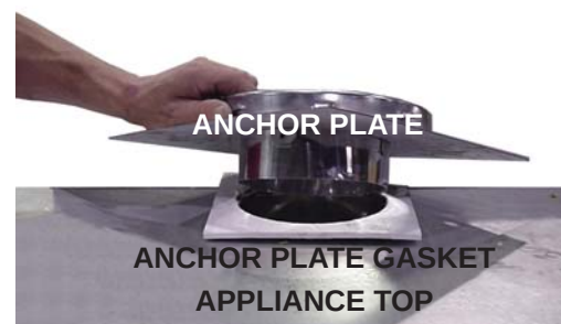
ANCHOR PLATE FOR A FACTORY BUILT CHIMNEY
