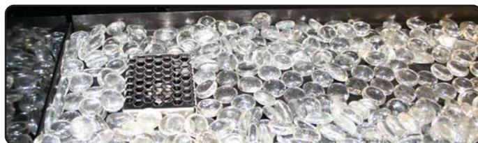
Figure 24.b Completed firestone installation
