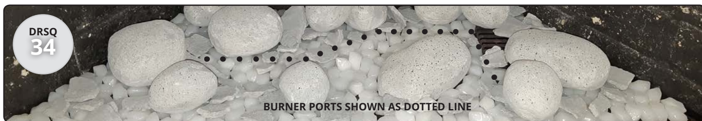
Figure 24.cc Completed Stone installation
