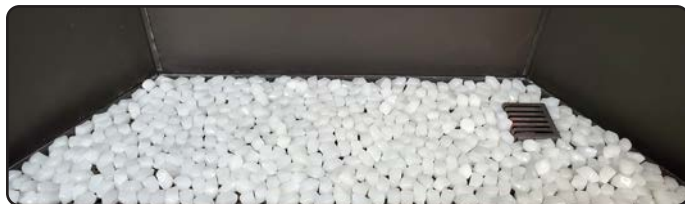
Figure 24.bb Completed firestone installation
