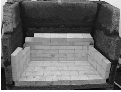
Figure 9. Firebrick Installation
