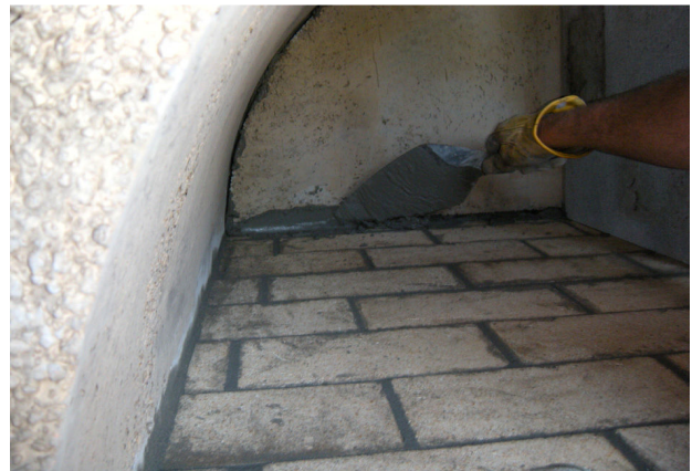
Figure 14. Mortar Inside Joints
