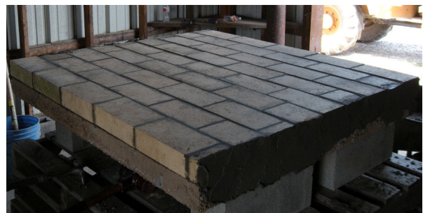
Figure 10. Install Firebrick on Baseplate
