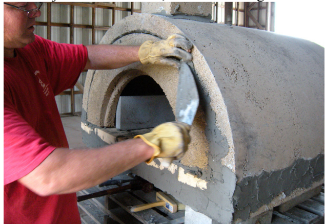
Figure 15. Install Front Wall
