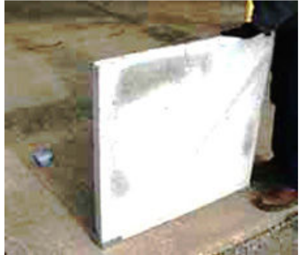
Figure 6. Place Back Panel in Bracket
