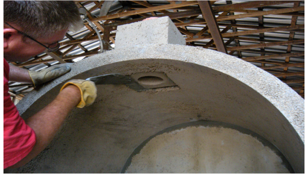
Figure 13. Mortar Chimney Inside of Oven
