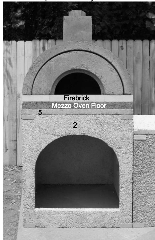
Completed Assembly with Oven
