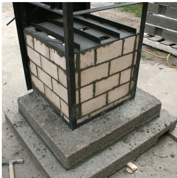
Figure 8. Firebox Completed
