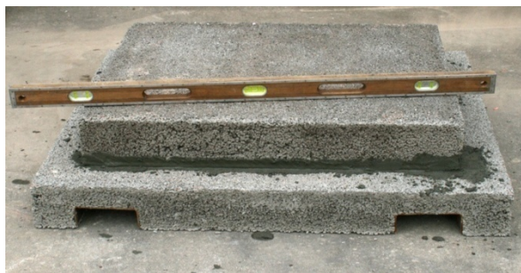
Figure 3. Set the Base Plate
