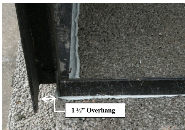
Figure 5. Provide Overhang at the Front
