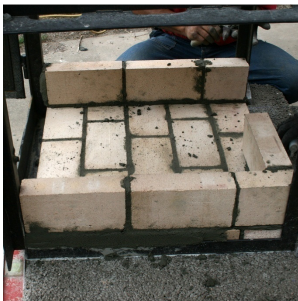
Figure 7. Install Brick Walls
