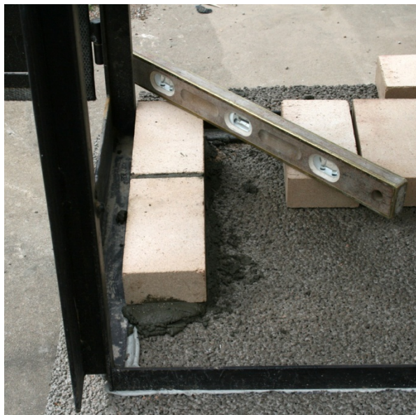
Figure 6. Lay Floor
