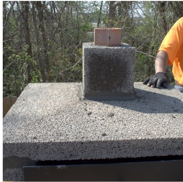
Figure 12. Add Chimney Section
