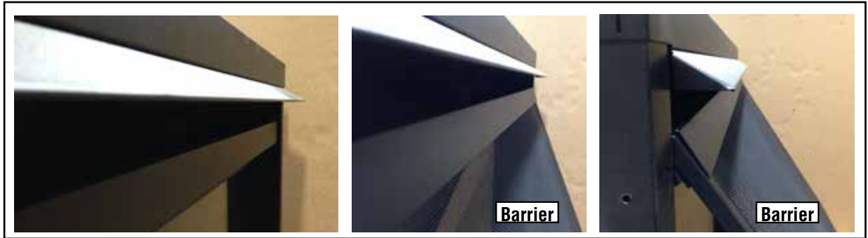
Figure 47A - Slide Barrier into Upper Trim Panel
