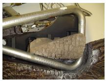
Figure 27A - Installing Charred Log Top View
