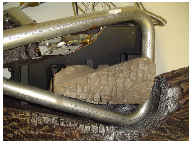
Figure 19A - Installing Charred Log Top View
